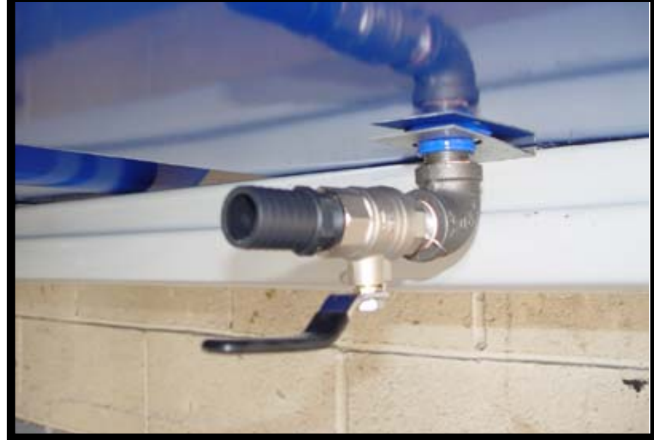
6 – Install hose connections on the bottom of the containers
