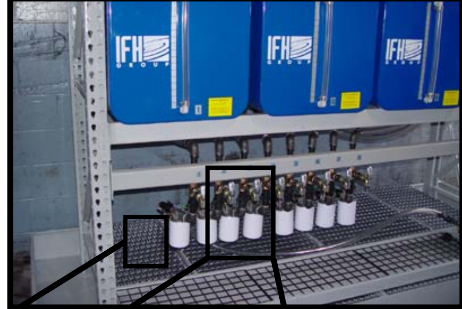
8 – If filtration was supplied, install the filter units
