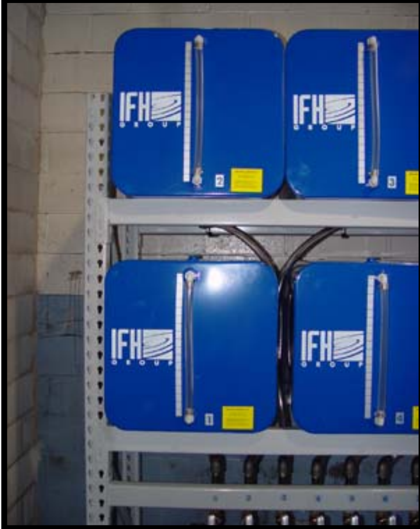
9 – Connect the hosing from the containers to the spigots
