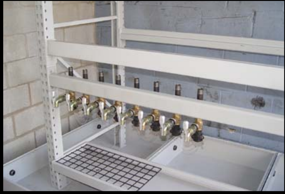
5 – Install oil spigots and drip tray
